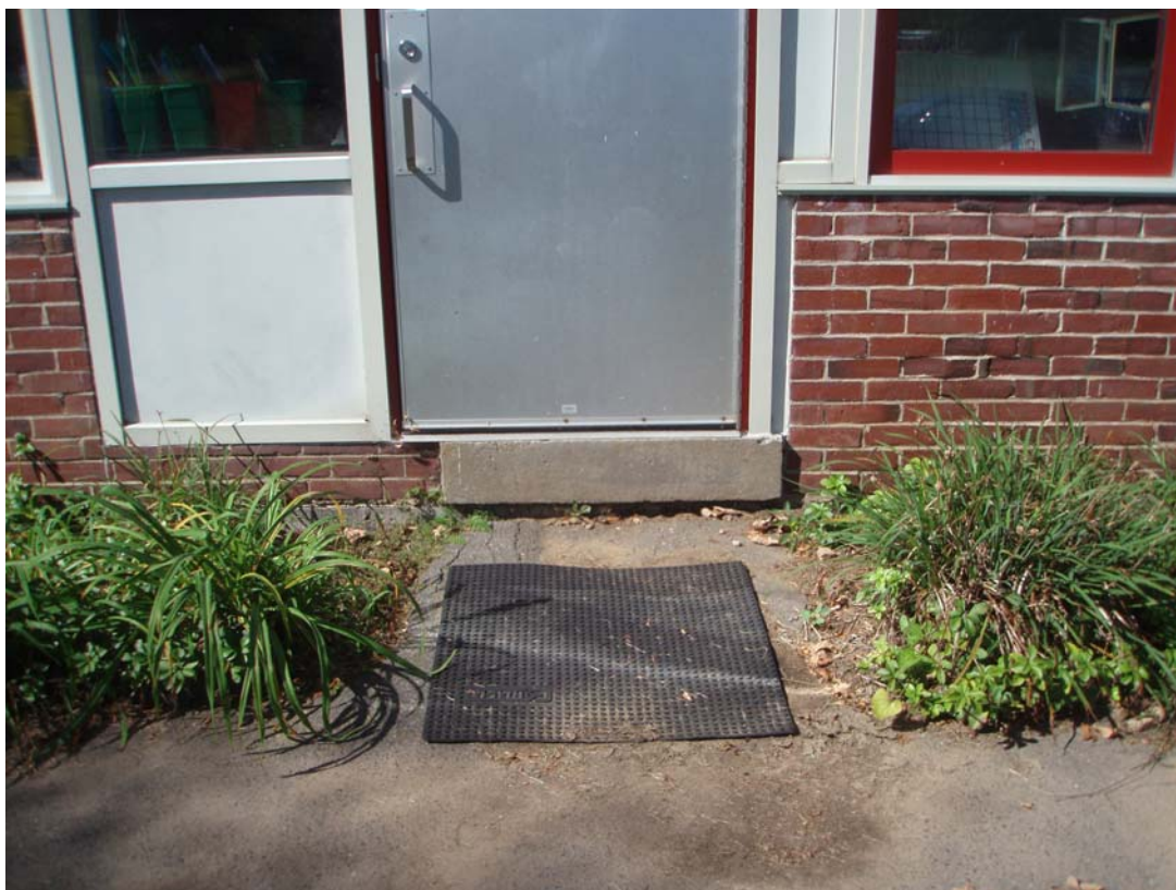
Picture 1.61 Some bathrooms are not compliant with MAAB accessibility standards Picture 1.62 A number of classroom exits are not wheelchair accessible
