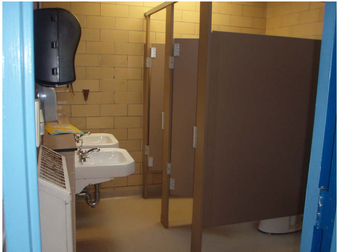
Picture 1.61 Some bathrooms are not compliant with MAAB accessibility standards Picture 1.62 A number of classroom exits are not wheelchair accessible
